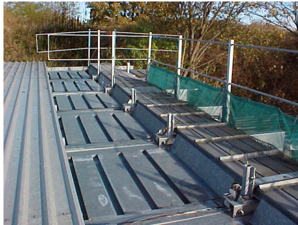
Plate 2: Main Components of purlin trolley system ( Jayeff's Leadguard )
