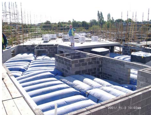
Plate 17: Configuration of air mats in domesticated housing sector (© Bison)
