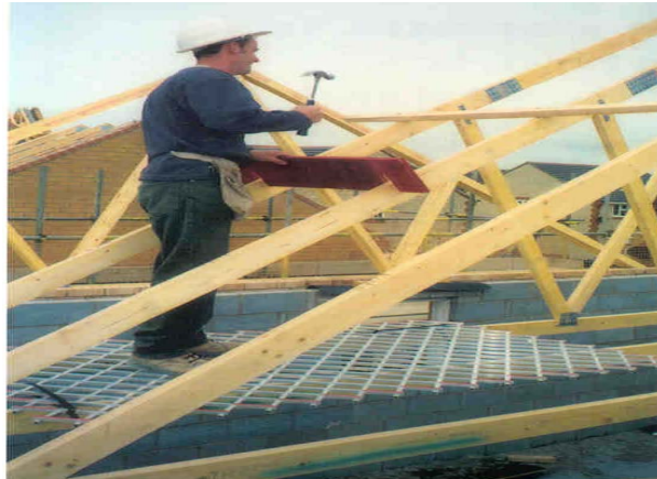
Plate 12: EAT set-up deck for use to first-fix trusses
