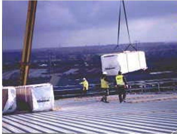
Plate 3: Loading roofing materials to safe zone on roof ( supplied by Rossway Dowd )
