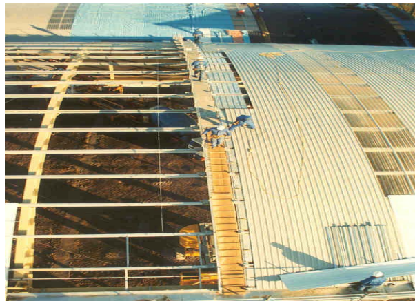
Plate 1: Purlin trolley system used on a curved roof ( courtesy of Jayeff Ltd )
