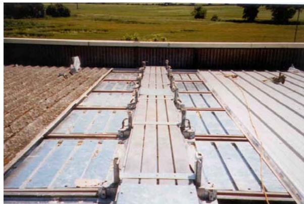
Plate 4: Modified purlin trolley in a roofing refurbishment situation. Note the old and new roofing covering. Edge protection should be provided under such circumstances.
