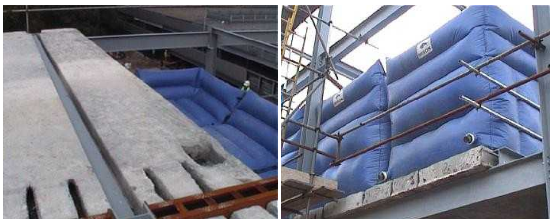
Plate 19: Parapet air-mat configuration in an industrial situation, providing cushioned edge protection and passive fall arrest (© Bison)
