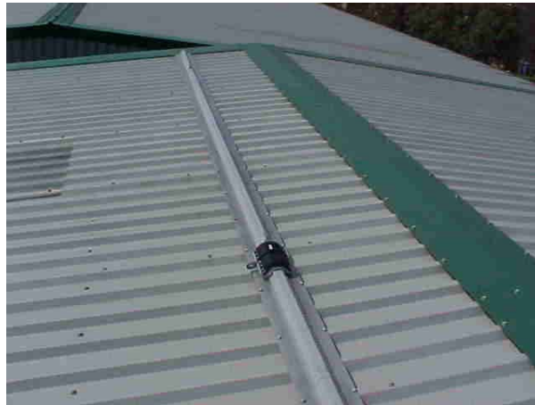
Plate 28: Typical track safety system attached to roof covering for arrest protection during roof maintenance works, showing the track and traveller ( courtesy of Saferidge )
