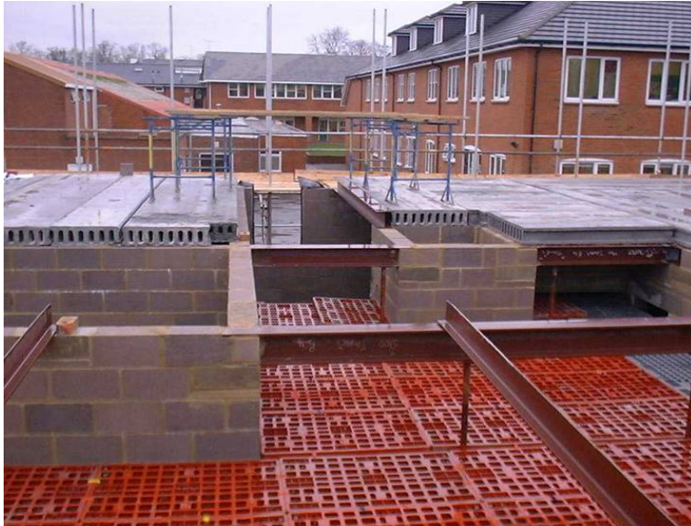
Plate 7: Typical PDS used in a domestic housing construction setting ( courtesy of Tarmac ) 6
