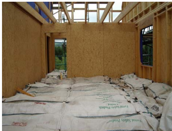
Plate 18: Soft-filled mats installation in domesticated housing ( Site visit, June 2003 )
