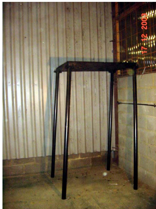
Plate 11: Standards leaning into corner to keep the first panel from falling over
