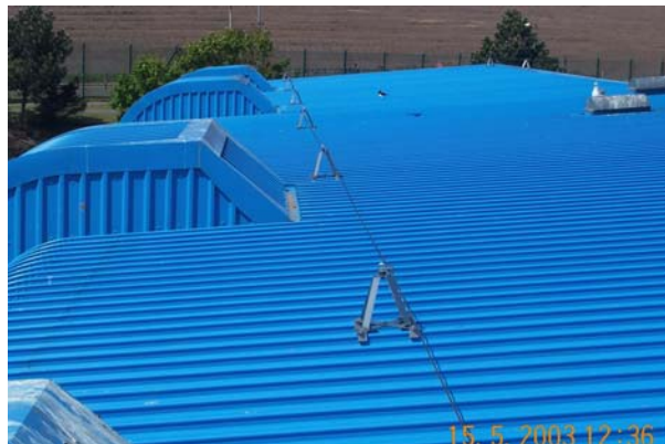
Plate 27: Typical cable system in-situ for arrest protection to operatives during roof maintenance, showing cable running through anchorage posts ( Taken during site visit to BNFL, May 2003 )
