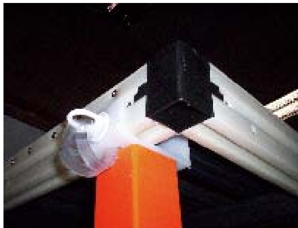
Plate 10: Pin arrangement connecting prop to decking panel ( courtesy of HL Plastics )
