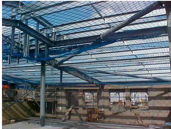
Plate 20: Safety nets in low-rise industrial construction setting. Netting positioned as close as is possible to the underside of the roof structure
