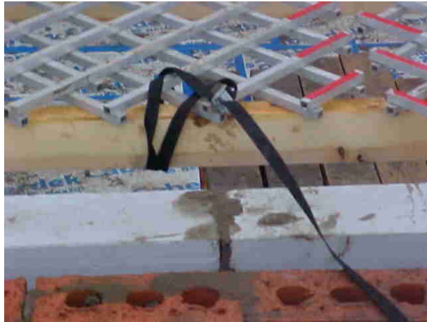
Plate 14: EAT deck fixed by the securing straps at each end
