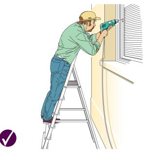
Figure 3a Correct - rungs facing work activity
