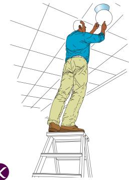
Figure 4b Incorrect - working from the top step with no handrail
