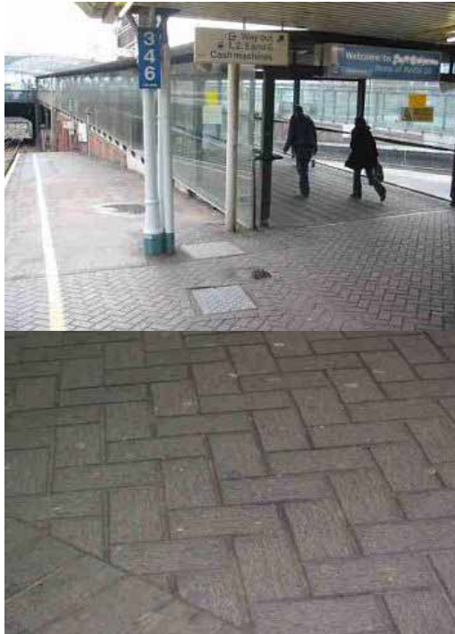
Ramped walkways after resurfacing.
