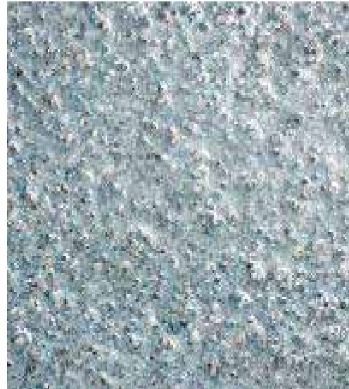
The finished floor with an even distribution of anti-slip treatment.
