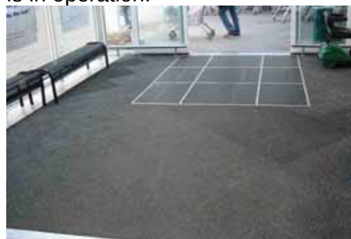
A store entrance following improvement work.
