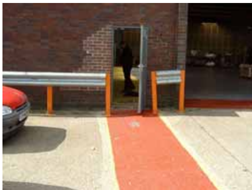
Pedestrian access route and painted vehicle access route floor.
