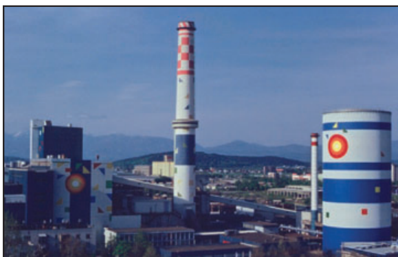
The TE-TOL plant
