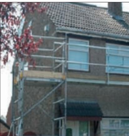
If a half platform is in use, a guard rail must be fitted, with toe-board, to prevent falling from the inside of the platform. At no time should operatives climb on the outside of the tower scaffold, particularly during erection and dismantling.
