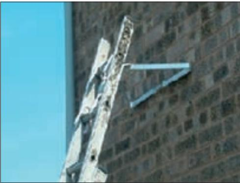
Ladders must only be used on firm level ground and must form an angle of approximately 75° to the horizontal, ie 1m out for each 4m of height. Such an angle minimises the potential for base slippage when in use. This angle is indicated on Class I ladders by a line or arrow on one stile, when this mark is vertical the ladder is at the correct angle.
