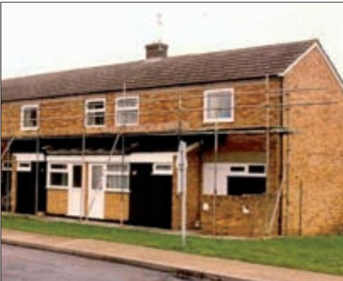
Any scaffolding encroaching onto a public road or walkway must only be erected after the issue of a local authority licence authorising such a structure. The fitting of reflective tape and/or lighting up to a height of 2.5 metres on the structure, to provide a hazard identification, is a requirement in such instances. The provision and fitting of such items should be carried out by the Supplier in compliance with the terms of the licence.
