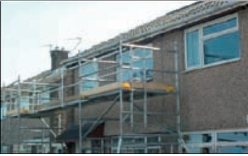
All mobile towers must be erected as shown in the Manufacturer's/Supplier's instructions, by a competent person. For example those trained to PASMA (Prefabricated Access Supplier's and Manufacturer's Association) or an equivalent standard.
