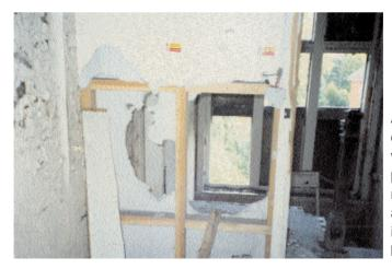
A severely damaged wall partition made of asbestos insulating board.
