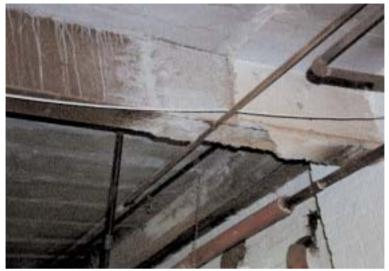
Steelwork coated with asbestos spray for fire protection. The photograph also shows a section of asbestos lagged pipework. The insulation on both has been partly removed.
