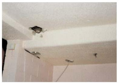
A ceiling coated with asbestos spray, which has been damaged by building work.
